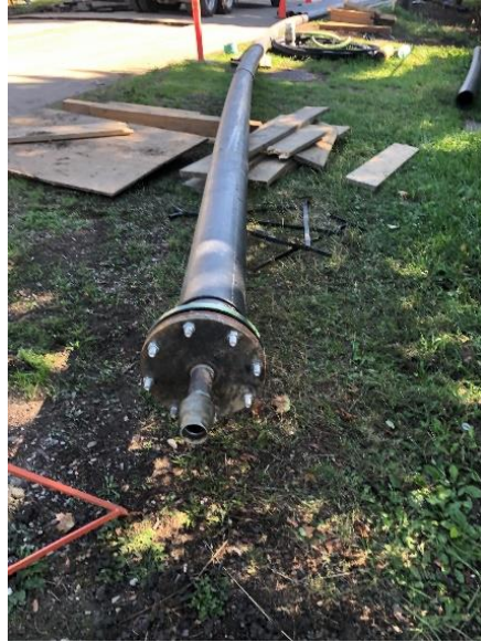
Figure 2 -Pressure tested pipe ready for installation.
